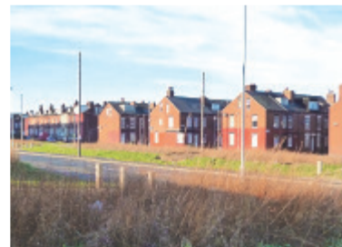
Before: derelict land left after demolition of poor-quality homes.
