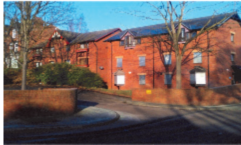
Umoja House, boarded up and awaiting refurbishment.
